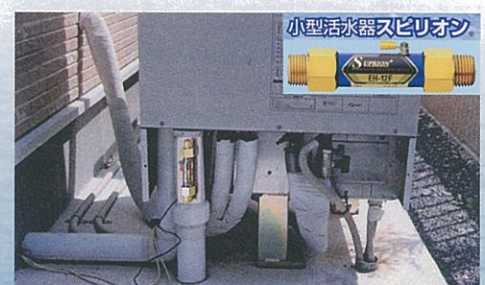
CO2 refrigerant applied Hot water boiler
